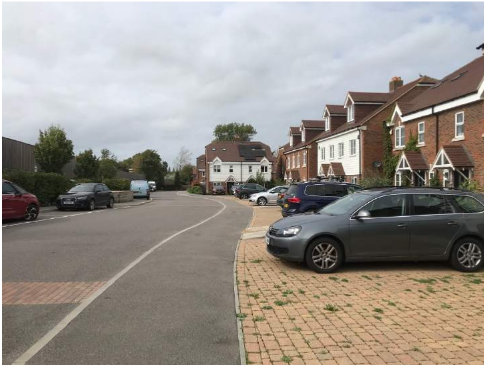
Above: The public realm of this cul-de-sac development is negatively impacted by the visual dominance of the car parking, either through the placement of on-street or front curtilage bays. Image credit: Deeper Green
