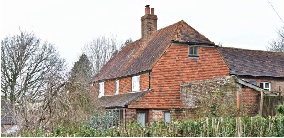
Above: An example of a traditional roof form, Oast House on the Catsfield Road. Image credit: Deeper Green
