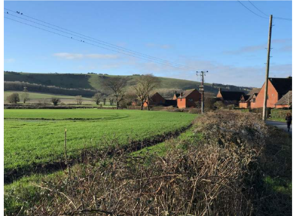
Above: An example of settlement edge development in Ringmer East Sussex. It underlines a successful built response to a landscape-dominated setting with careful attention to building placement and form as well as choice of materials. Image credit: Deeper Green
