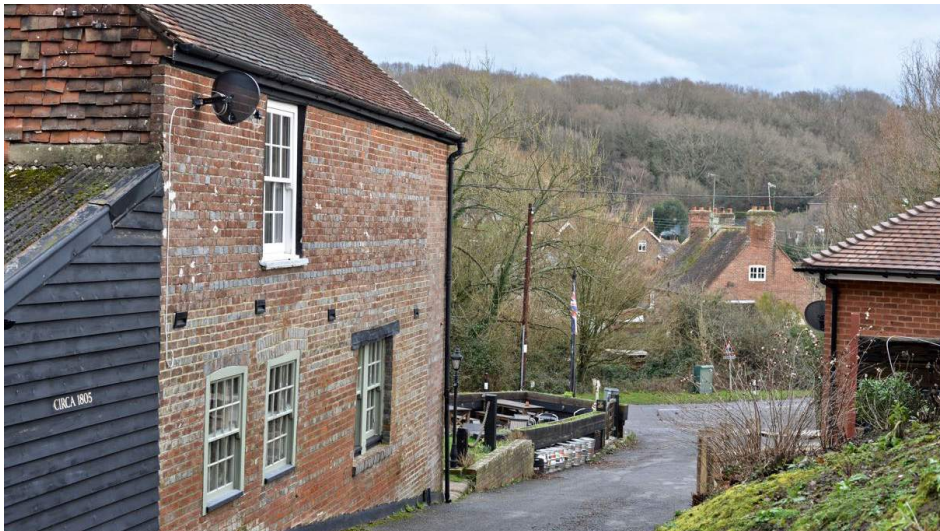
Above: The Plough Inn exemplifies the use of brick (here with contrasting bands of grey brick), plain clay roof tiles, hung clay tiles and a timber clad out-building. Image credit: Deeper Green
