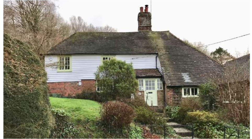
Above: Many of the older cottages have a brick ground storey and timber clad upper storey as in this example on Sampson's Lane. Image credit: Deeper Green
