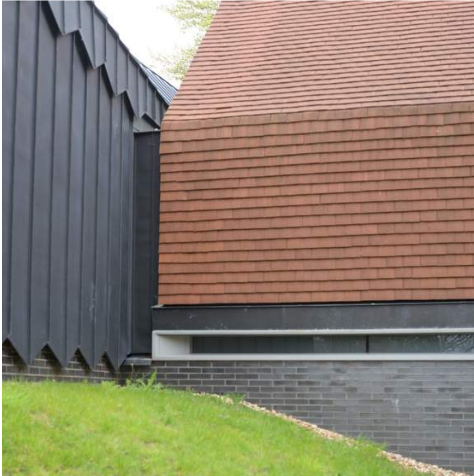
Above: Juxtaposing traditional and contemporary forms of materials with plain clay tiles and black patinated zinc. The Ditchling Museum by Adam Richards Architects. Image © Deeper Green
